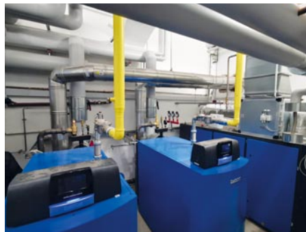
Energiezentrale, Herder-Gymnasium, Forchheim
